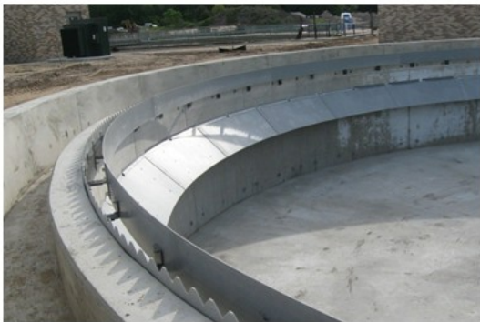
Weirs, Scum Baffles & Density Current Baffles
